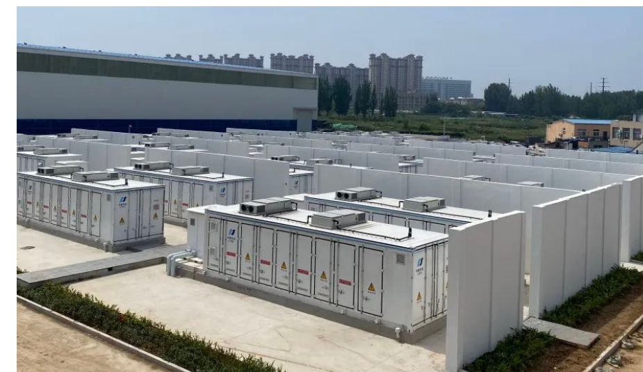
● The world's first 100MW energy storage power station which adopts the HV series-connected direct-hanging energy storage technology
